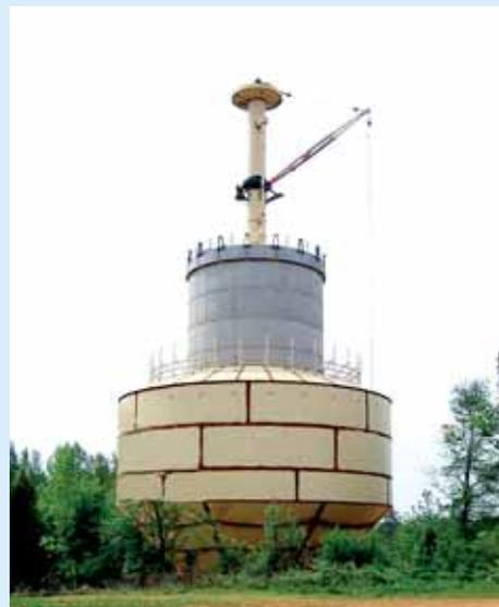
The City's fifth elevated water storage tank is currently under construction at the intersection of Heckle Boulevard and Rawlinson Road. The photo to the left shows the bowl situated at the base of the tower, positioned to be raised to the top after it is painted. The tank is expected to be in operation by August 2007.
