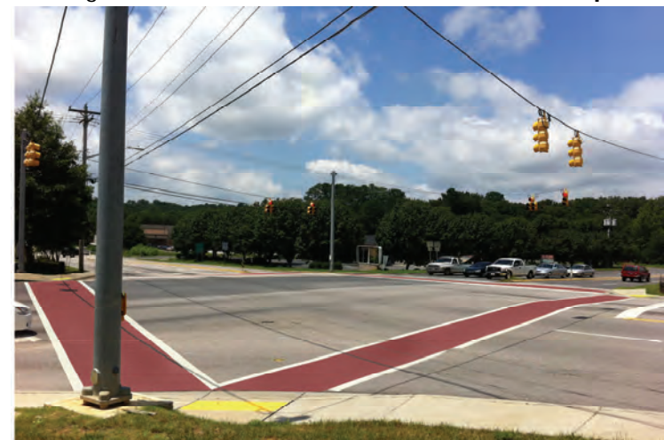
Recommended crosswalk upgrades
