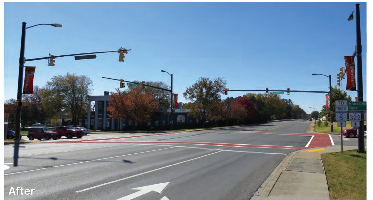
Main Street/Cherry Road Intersection with Upgrades
