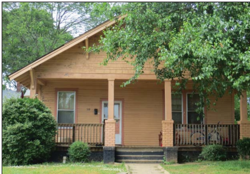
516 Hagins Street- 2015 Survey
