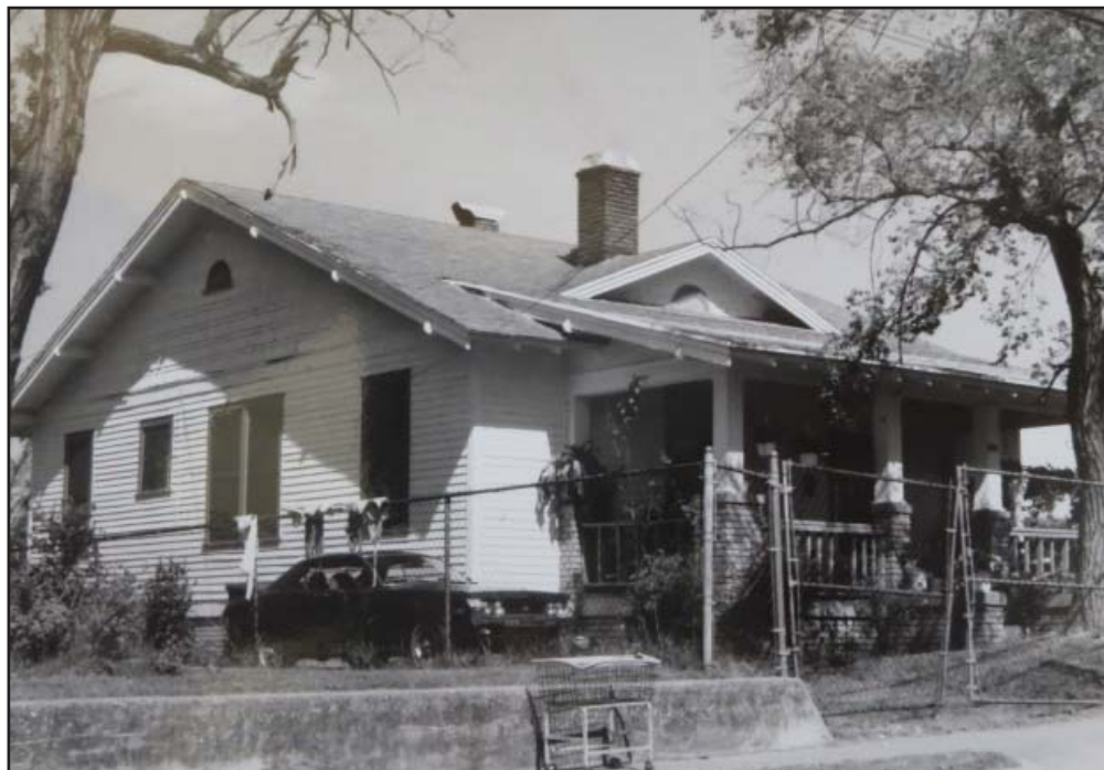
510 Hagins Street- 1988 Survey
