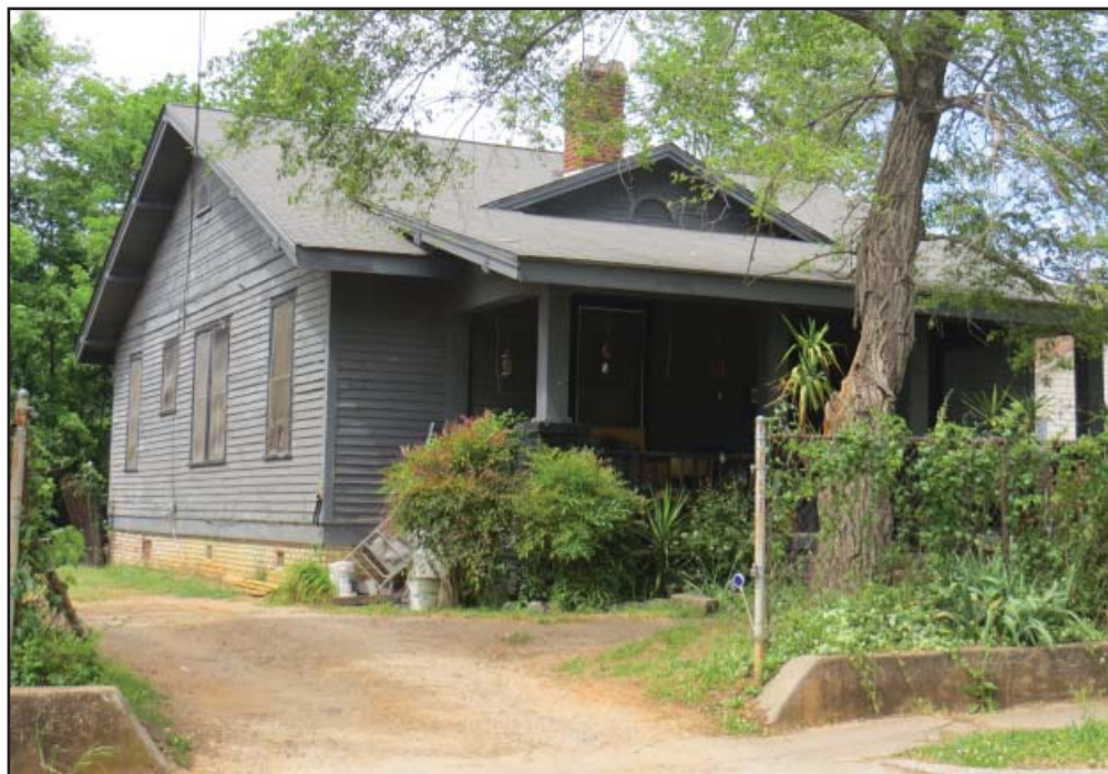
510 Hagins Street- 2015 Survey
