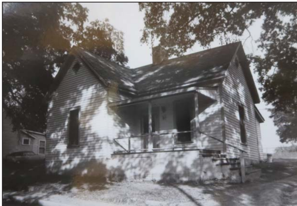
72 Reynolds Street- 1988 Survey
