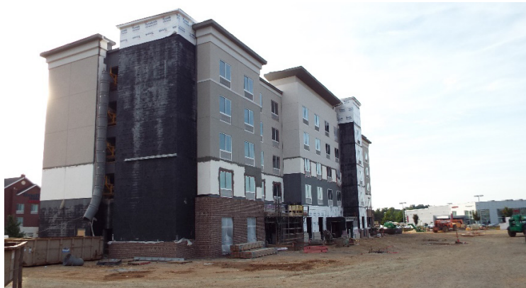
Fairfield Inn Hotel on Galleria Blvd. in Construction
