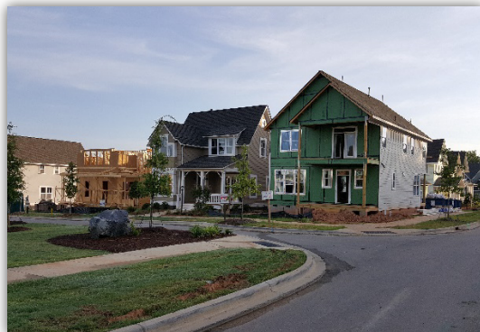
Riverwalk New Home Construction
