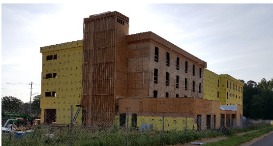
Home2Suites Hotel at 1285 Old Springdale Rd.
