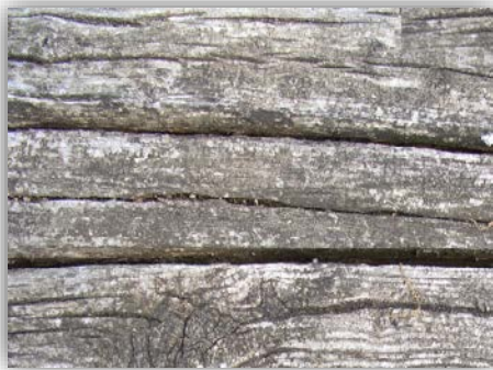
SIDING THAT COULD BE CONSIDERED FOR REPLACEMENT
