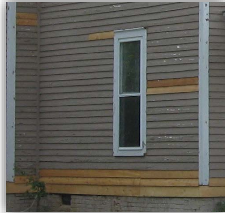
PROPER SIDING REPAIRS
