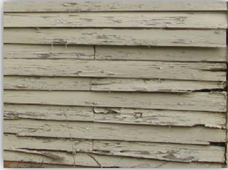
SIDING THAT COULD BE CONSIDERED FOR REPLACEMENT
