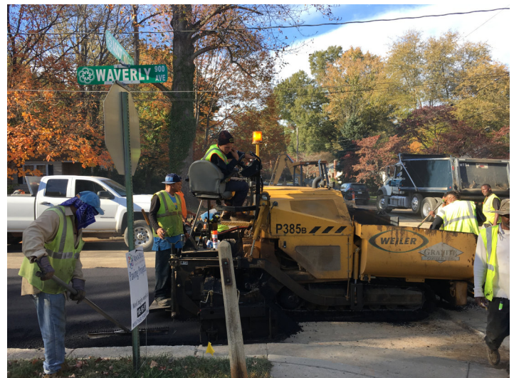
City crews repaving roads
