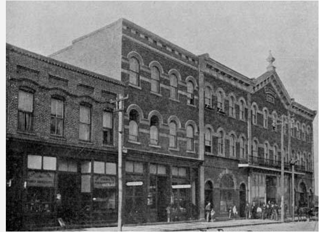
Roddey Building East Main Street, 1895
