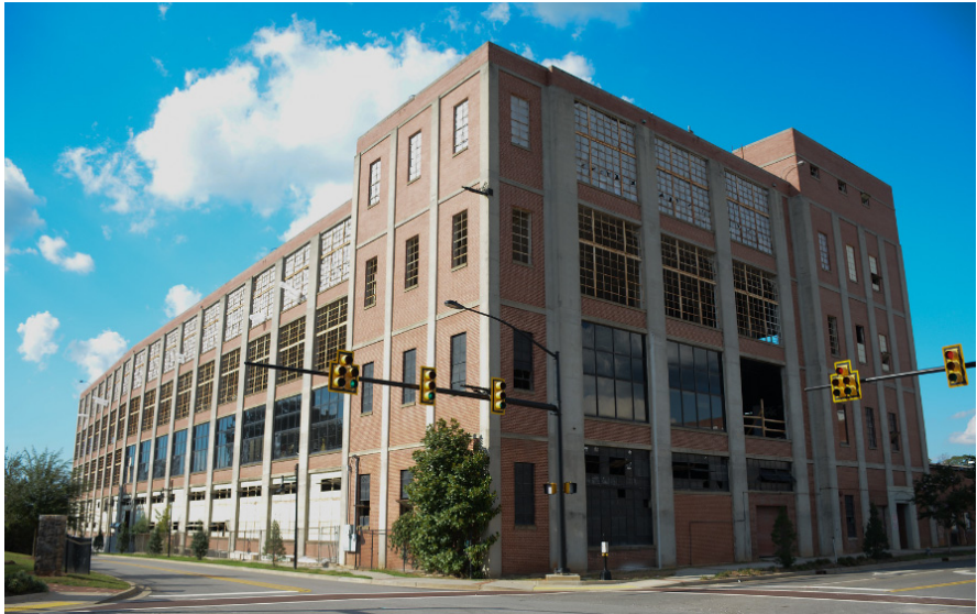
The Lowenstein Building (2018)
