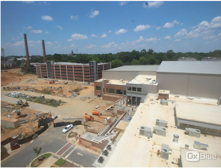
Construction continues on the University Center site.
