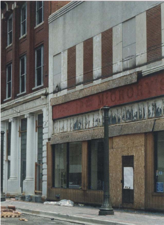
1990s (mall demolition)
