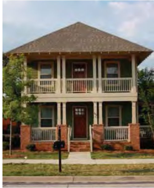
YES: Trim shown on stacked flat duplex façade with hardboard and brick materials.
