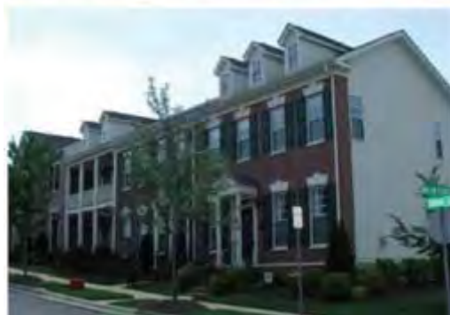
NO: Returns, or changing the material around the corner - in this case from brick to siding - looks incomplete
