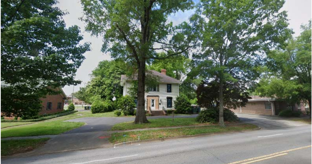
View of front façade & driveway (Google street view – 2019)
