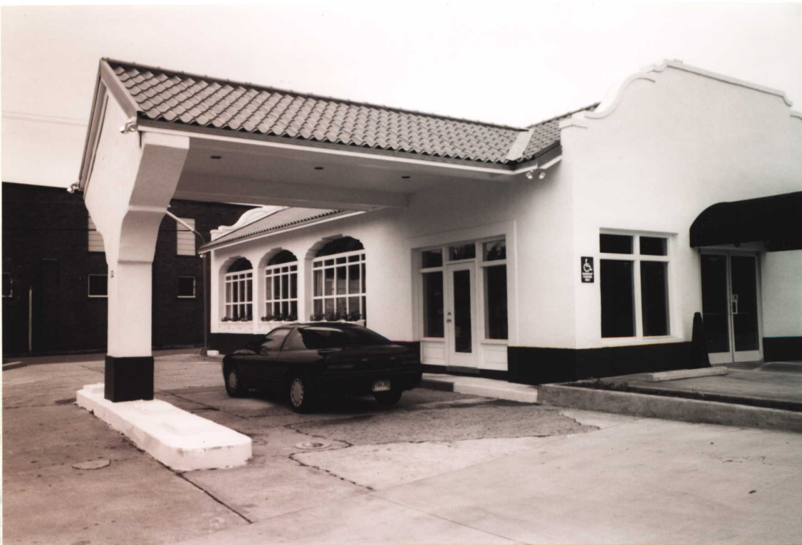
View of East Elevation
