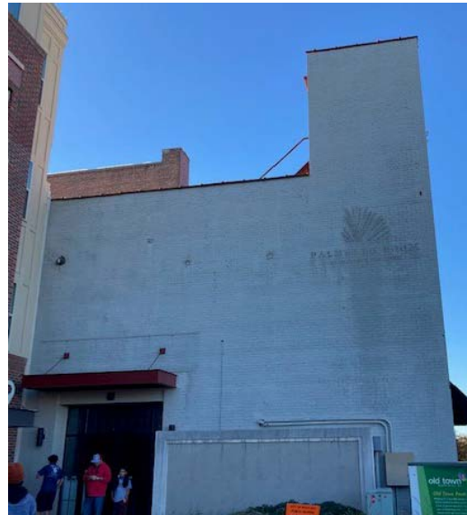
East White Street façade
