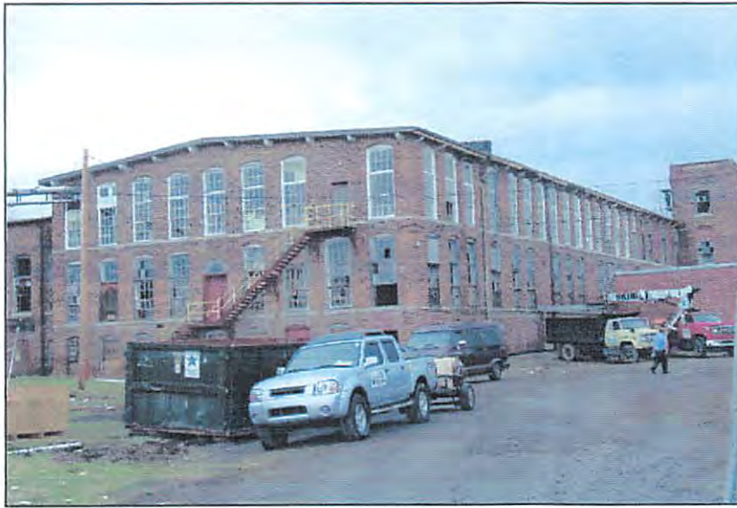
Highland Park Mill, No. 2, formerly Standard Mill (NR 1992)
