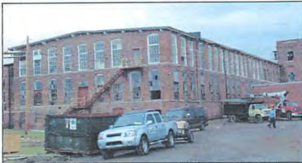
Highland Park Mill (NR 1992), renovations in 2004
