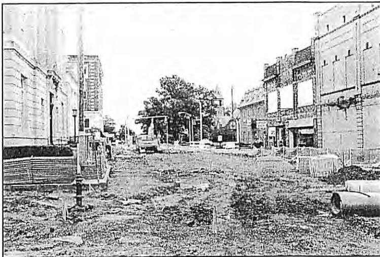
Removing Town Center Mall
