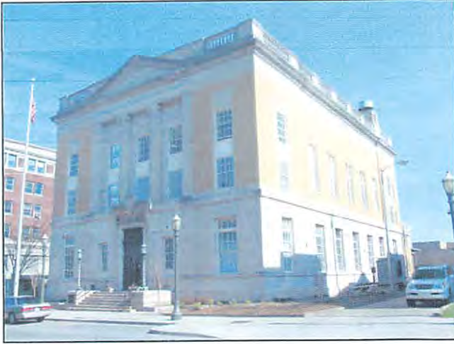
1932 Post Office and Courthouse (0201, NR 1986)
