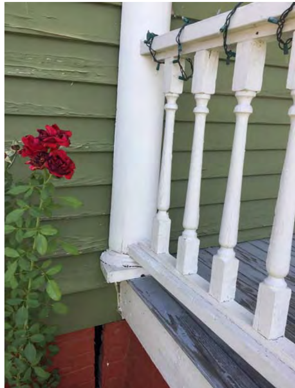
Left rear corner
