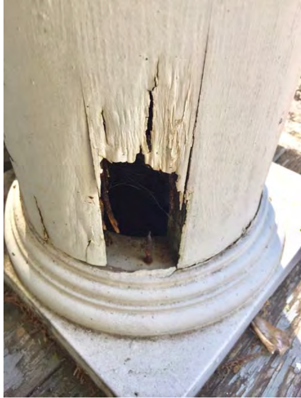
Immediate right of front steps
