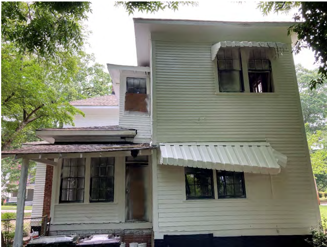
Rear façade – all proposed to be replaced
