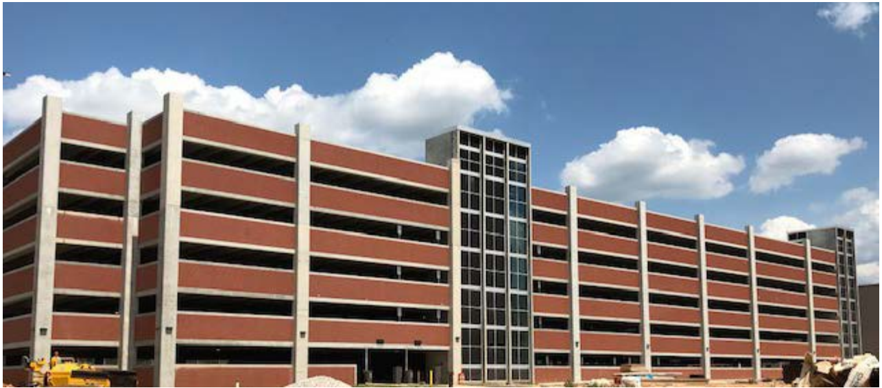
Parking Deck A completed in FY2020 at University Center.
