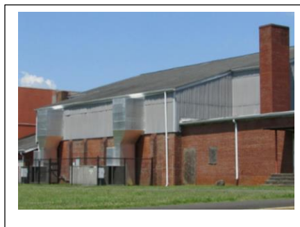
Figure 52. 1935 gym and assembly hall at Emmett Scott, 1936 image and current photograph. The Evening Herald Apr. 7, 1936, p5
