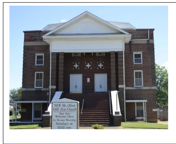
Figure 44. New Mt. Olivet AME Zion Church, current image from survey.
