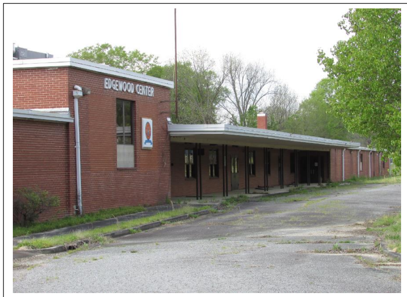
Figure 35. Edgewood Elementary School, current image from survey.
