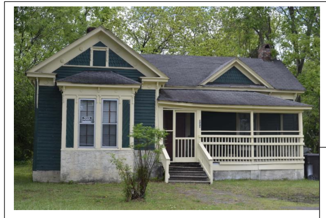
Figure 42. Excellent Queen Anne Victorian style at 234 Pond Street (#234) and at 1069 Flint Hill Street (#4602)
