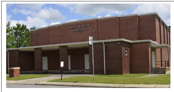
Figure 36. Emmett Scott High School Gymnasium, current image from survey.
