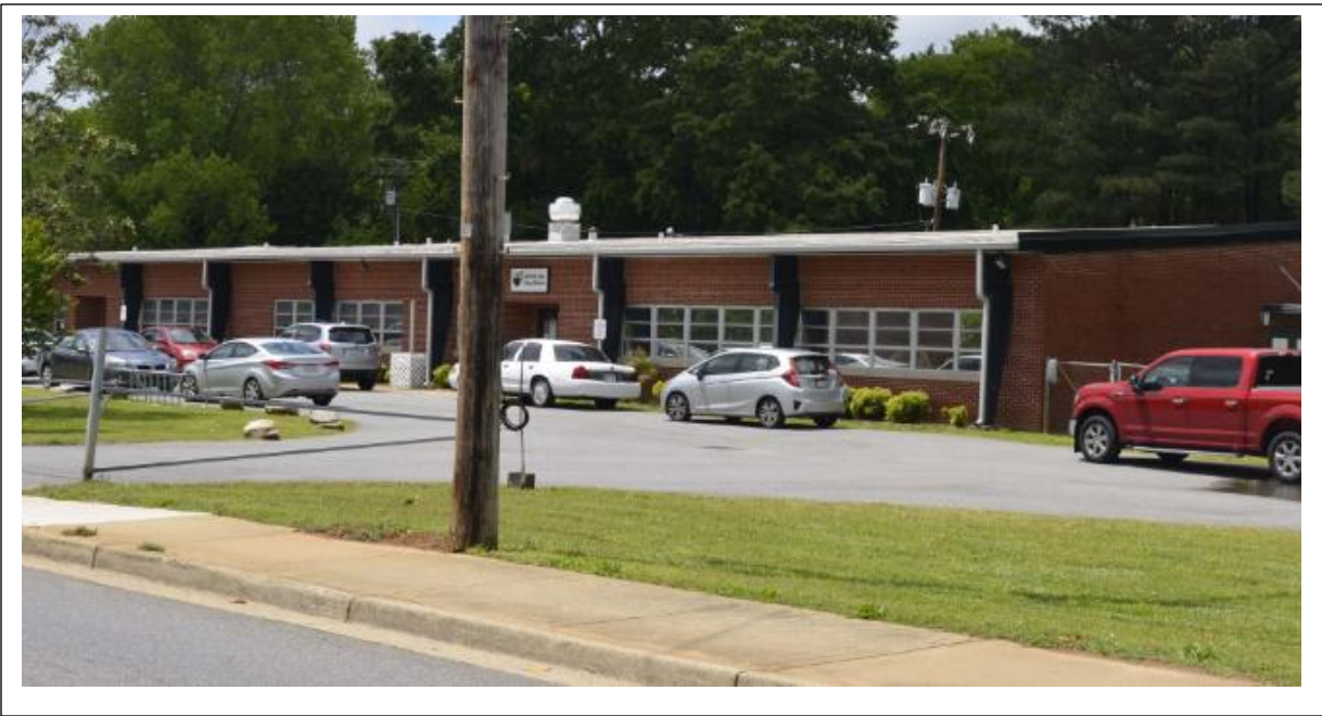
Figure 37. Bannon Hall, current image from survey.
