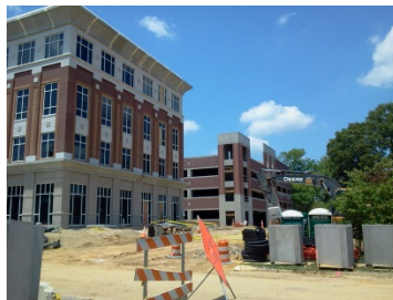
Old Town Professional Building and Parking Deck
