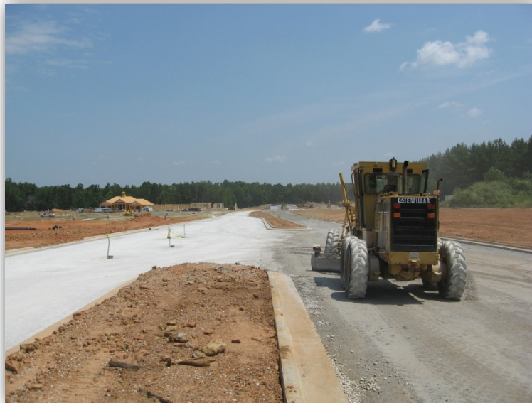
Extension of Galleria Blvd.
