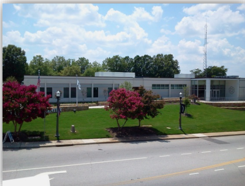
Rock Hill Law Center Addition
