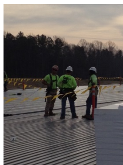
Inspections of roof at Exel Warehouse
