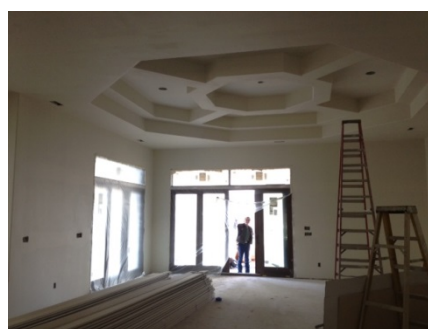
Rough-in inspections at new home in Laurel Creek
